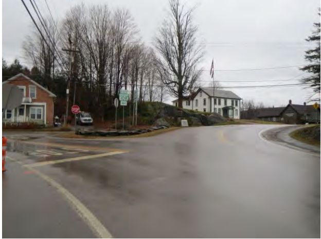
Lack of pedestrian accommodations and clear right-of-way make maneuvering this intersection confusing and unsafe
